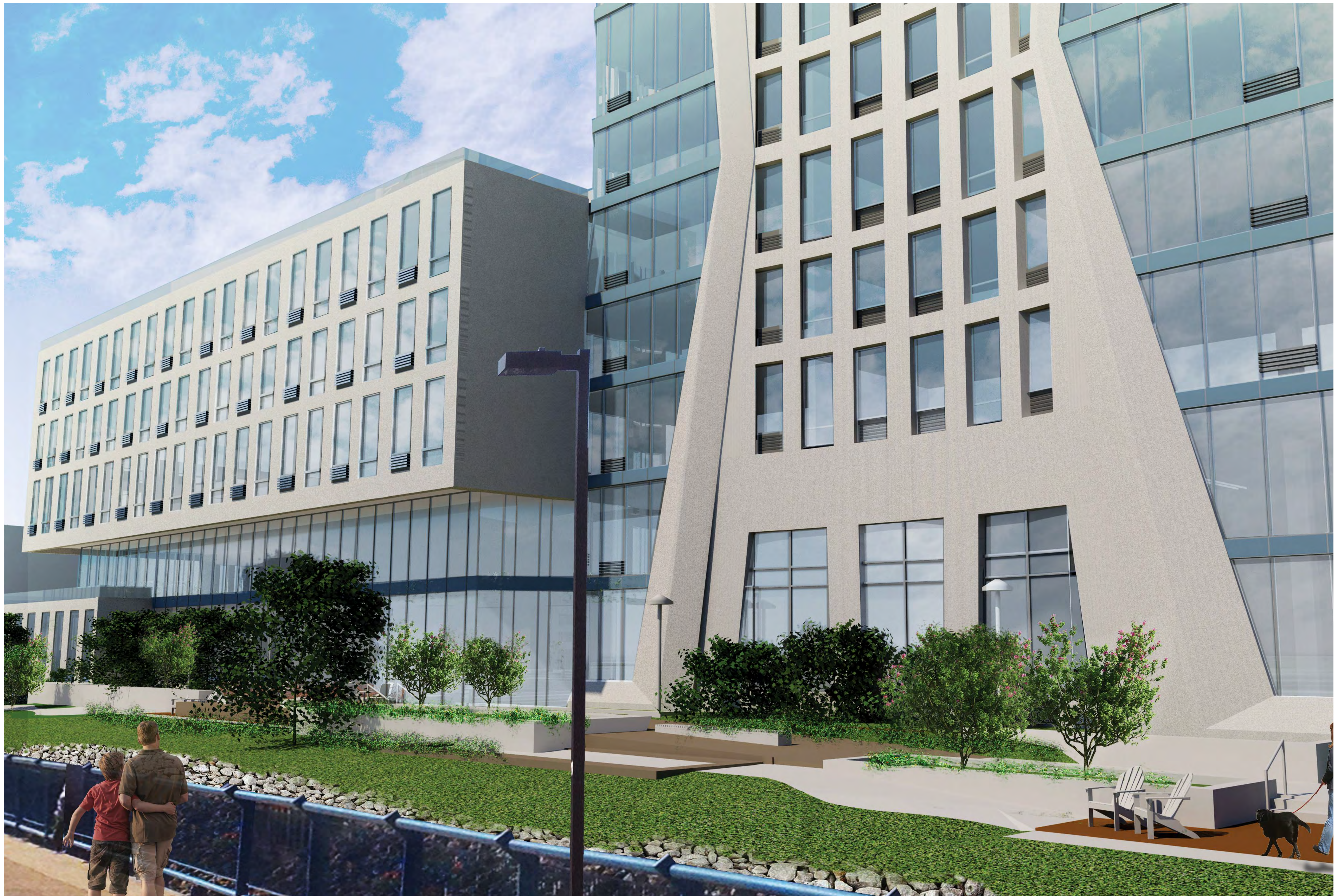
VIEW OF THE EASTERN ELEVATION FROM THE WATERFRONT WALKWAY
